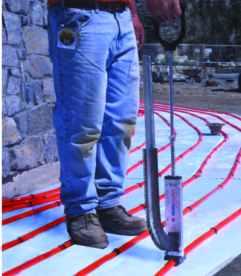
PEX tubing is stapled down in preparation for a cement pour at the Village Gondola terminal (above) as Xcel journeyman Art Moreno does a pre-fire inspection at Mammoth Center (below).
