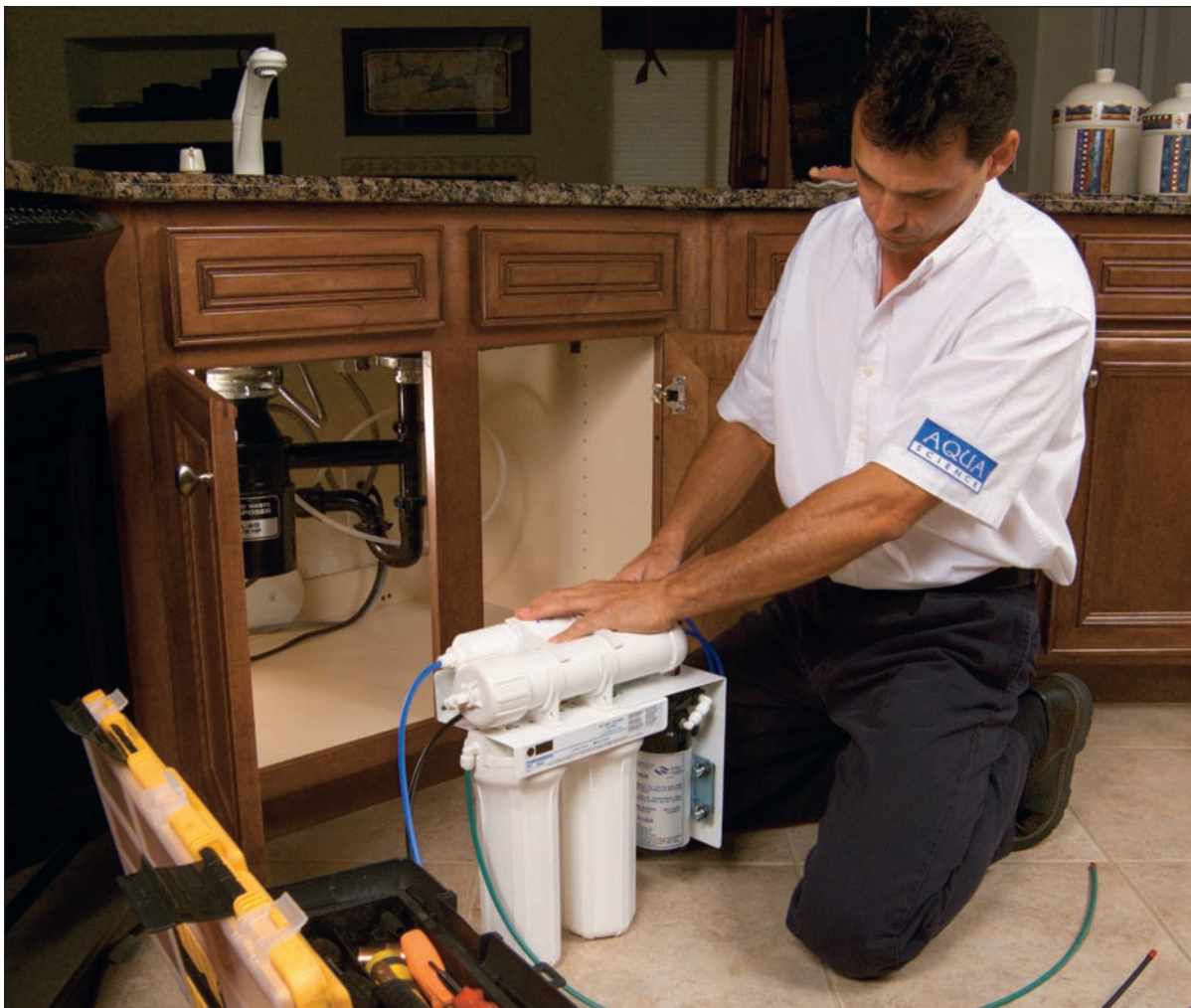
A zero waste reverse osmosis unit is prepared for installation.
