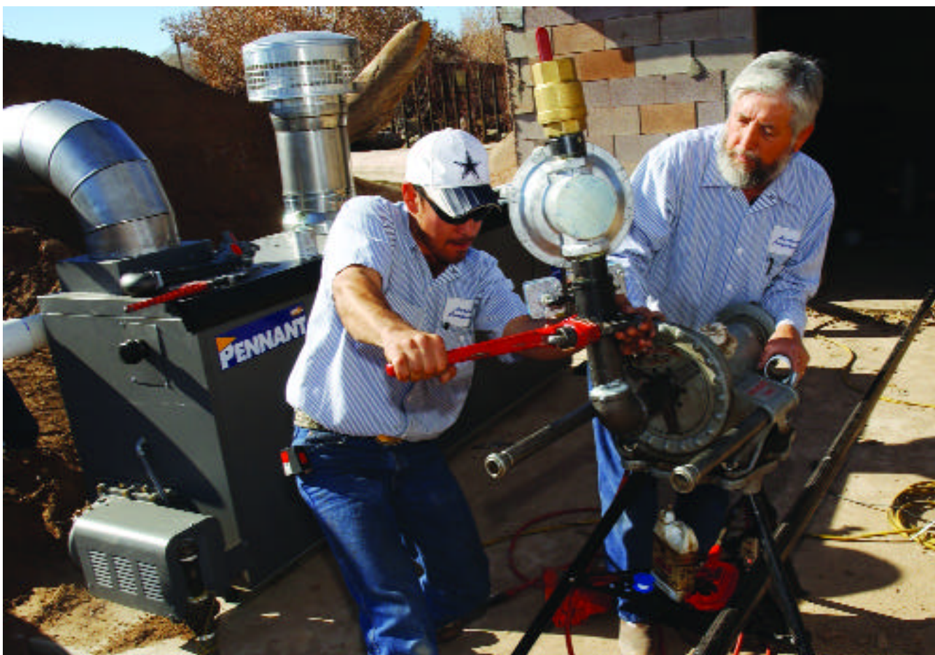
Aardvark Co. Inc.'s Juan Carlos Grijalva-Cervantes, apprentice, and Socorro Sotelo, master plumber, pipe gas to the boiler/water heater.
