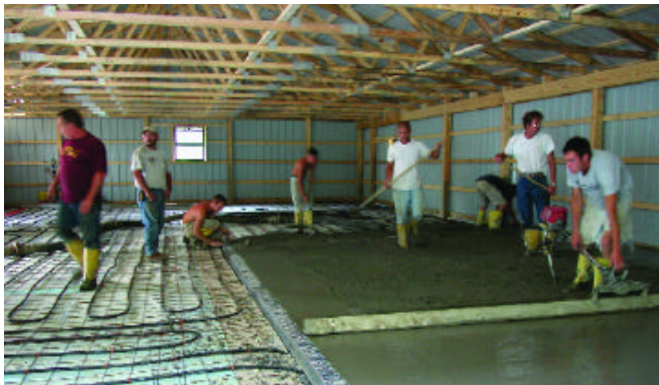
To keep costs down, Rehabitat’s regular volunteers took a crash course in radiant and helped install the system.
