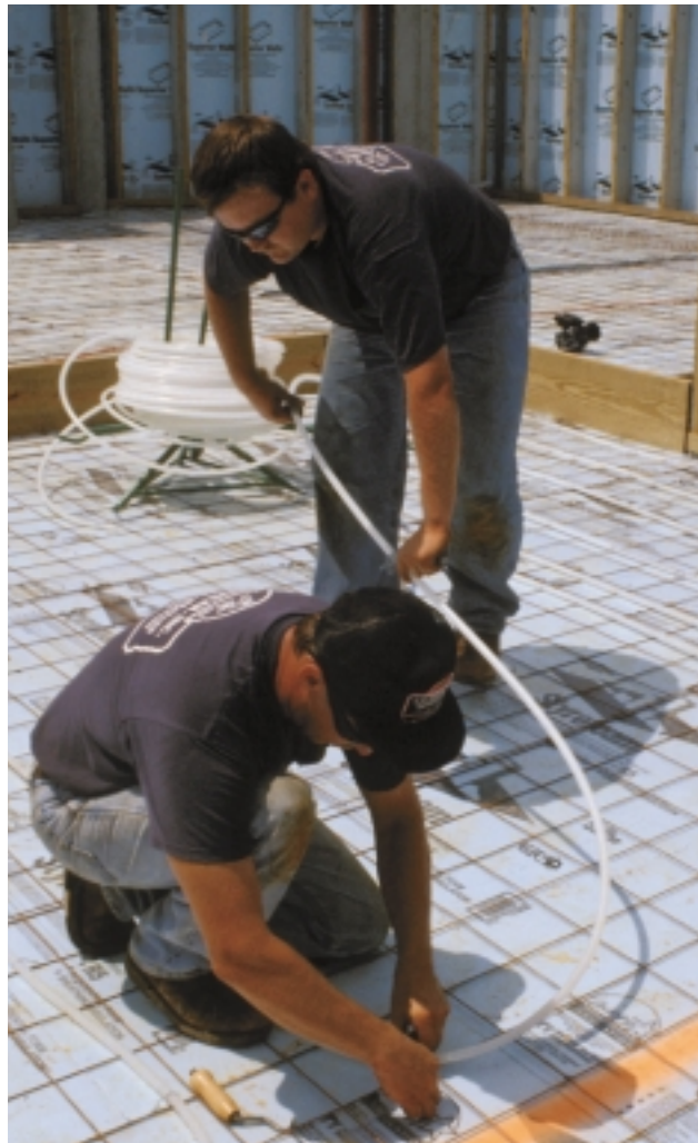
The most common method of installing radiant heat in basement slabs or slab-on-grade foundations is to attach the tubing to a wire grid.
