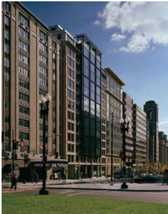
The Alta at Thomas Circle is an “official” (see sidebar, next page) 13 stories tall, with a penthouse and a five-level, below-grade parking garage.
