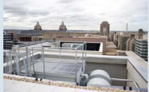
The Washington, D.C., skyline from the penthouse atop The Alta at Thomas Circle.
