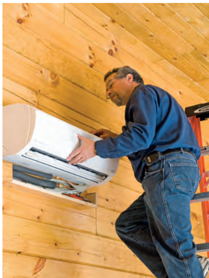
Dave Yates installs backup Fujitsu minisplit heat pumps, which also provide air-conditioning for interior garage spaces.
