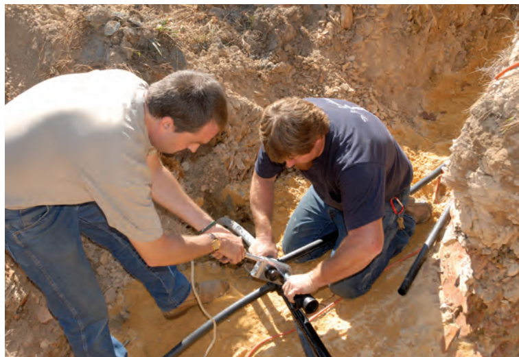
Fred Umble of Creative Energy (left) hot-fuses geothermal pipe connections at one of the three well-heads.
