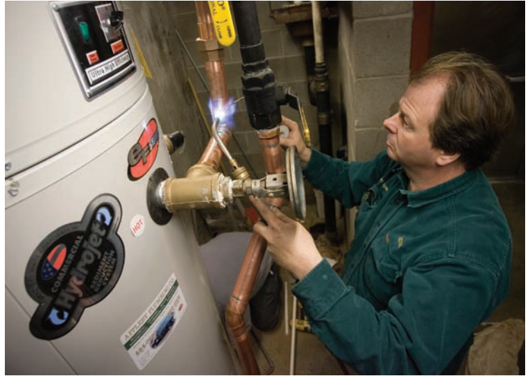
Chuck Appleby solders a joint (safety glasses removed for the photo).
