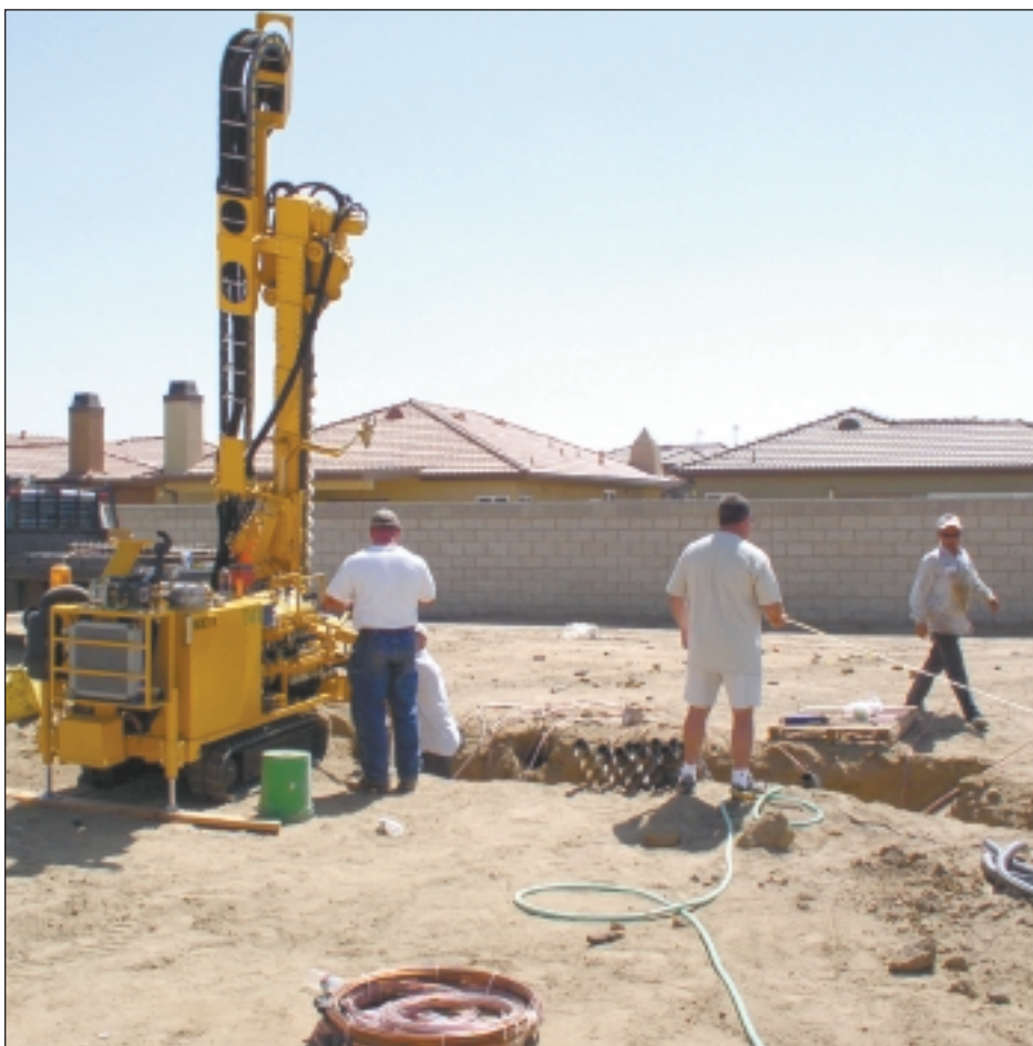
Earth loop installations need to be at least 50 feet away from a water well.
