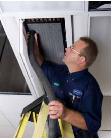
Alex Hof, a service technician with Wellington Controls in Guelph, Ontario cleaning the chilled beam coil and calibrating the temperature sensor for the supply water to the chilled beam.
