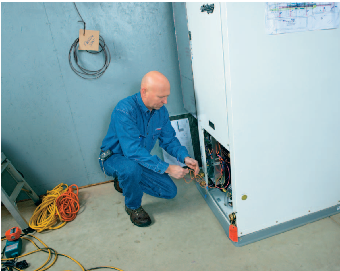
Jeff Persons of Geo Source One reviews wiring connections that will link the WaterFurnace Synergy III system to the multiple tasks for forced air and radiant heating loads it will handle. Photo courtesy of WaterFurnace.
