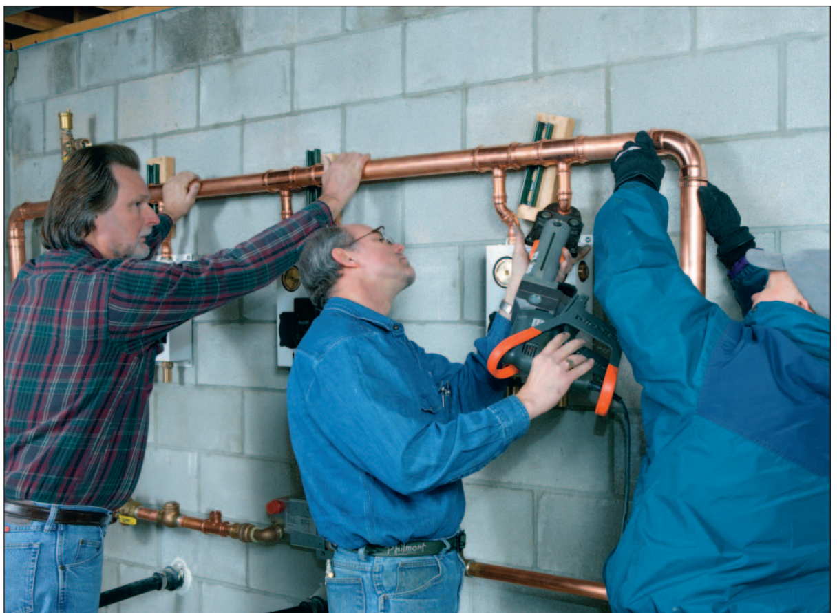
Teamwork to maintain all connections in their correct position allows Ron Whaley of Geo Source One to make quick work of over 60 copper-to-copper fittings on a massive primary-secondary geothermal pumping manifold. Geo Source One prefers the Pro-Press system for this work. Photo courtesy of WaterFurnace.
