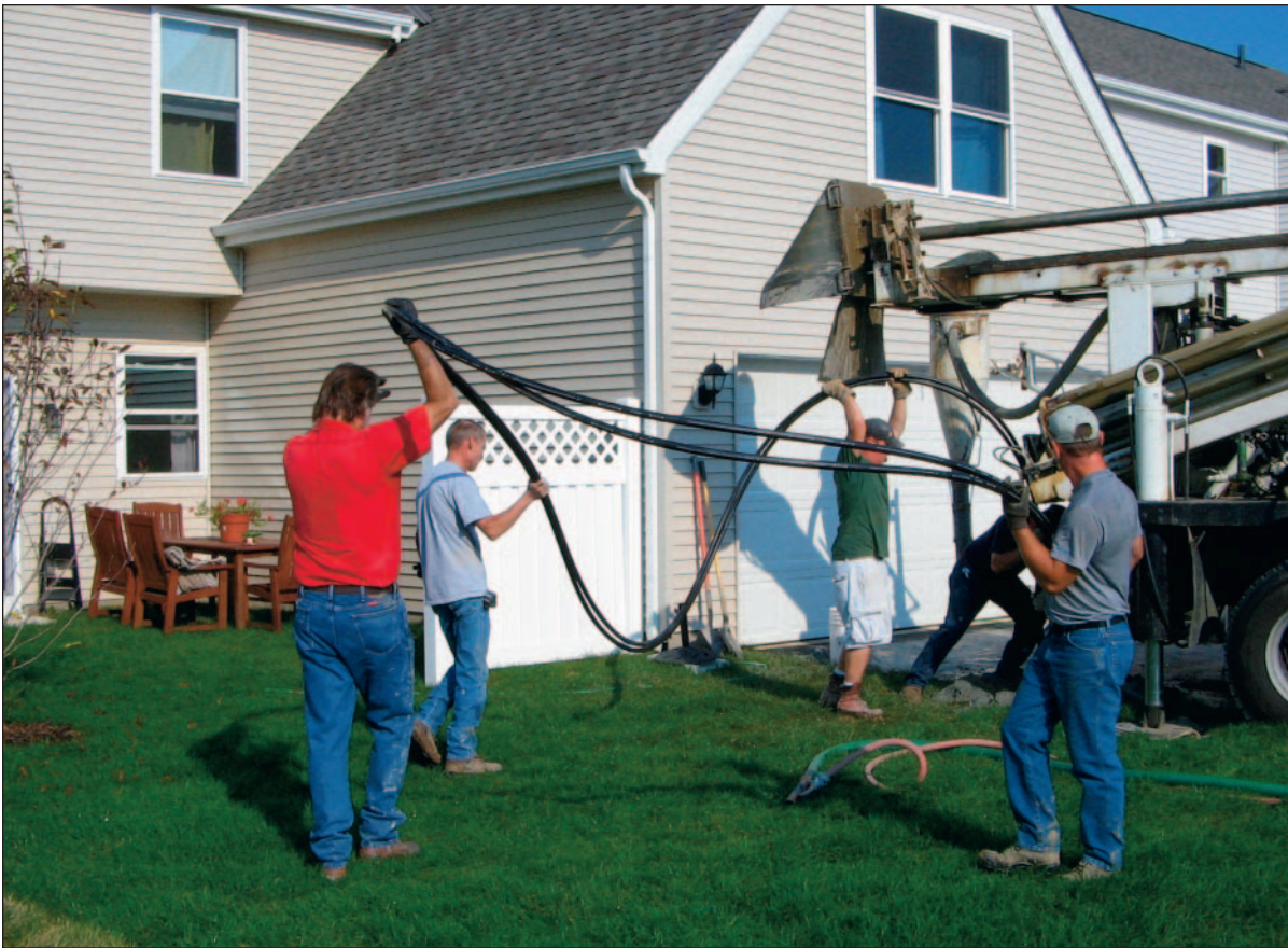
A crew installs a 150-foot polyethylene vertical loop line into a completed vertical heat exchanger well. Photo courtesy of WaterFurnace.
