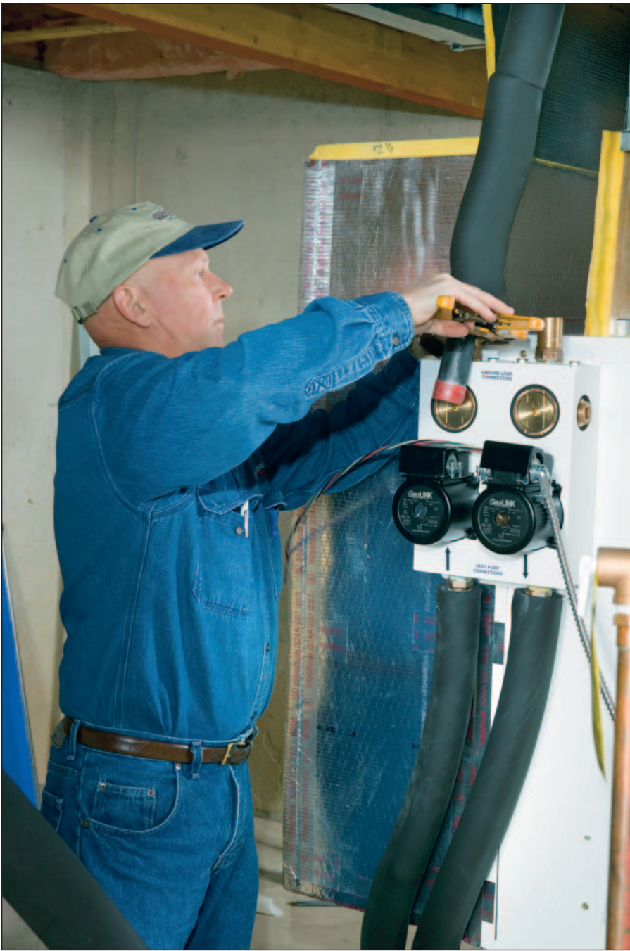
Jeff Persons of Geo Source One trims the polyethylene loop manifold lines prior to connecting to the geothermal loop "flow center" pump pack. Photo courtesy of WaterFurnace.
