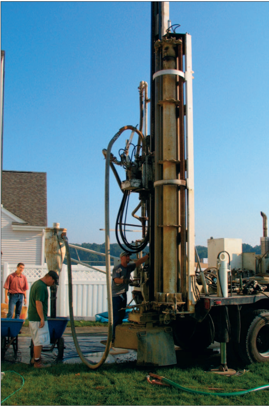
A drilling crew from Yoder Drilling and Geothermal sets up and drills the first of three 150-foot vertical heat exchange wells at a job in New Albany, Ohio. Photo courtesy of WaterFurnace.
