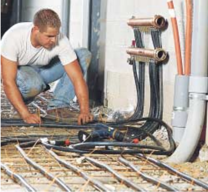
EPDM synthetic rubber "Onix" tubing is durable and flexible.
