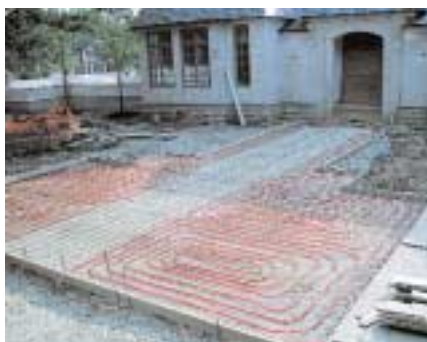
A snowmelt system (shown here, during and after) eliminates shoveling, scraping, salts and chemicals.
