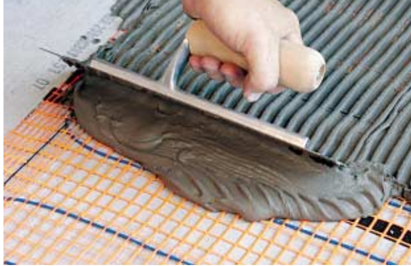
Thinset mortar is applied directly onto SunTouch electric mat.
