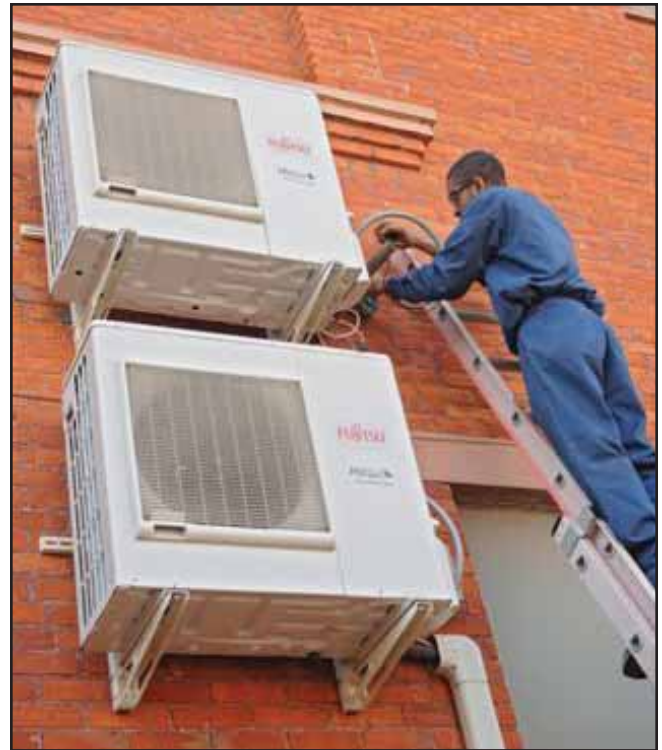
FIGURE 2. Wiring the wall-hung outdoor units.
