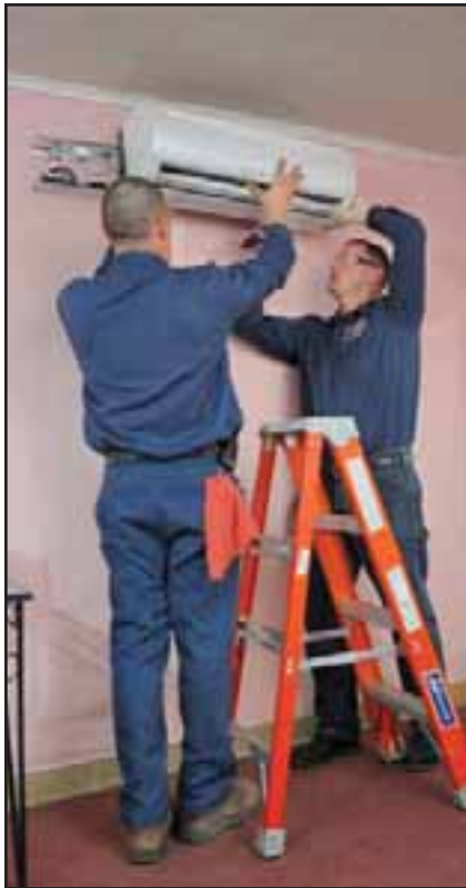
FIGURE 3. Installation of an indoor wall-hung evaporator.
