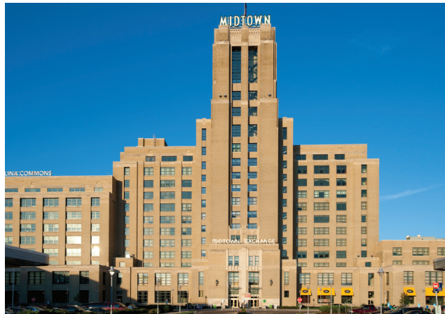
Midtown Exchange is the second-largest building in Minnesota, trailing only Mall of America.
