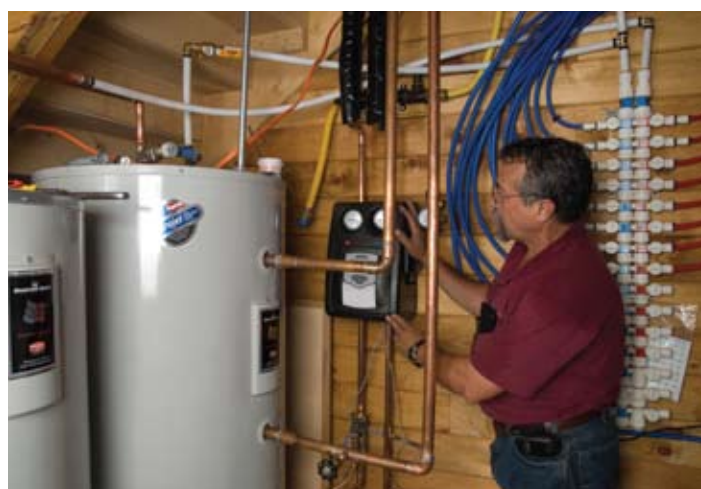
Dave Yates observes operation of the Oventrop solar pump station.
