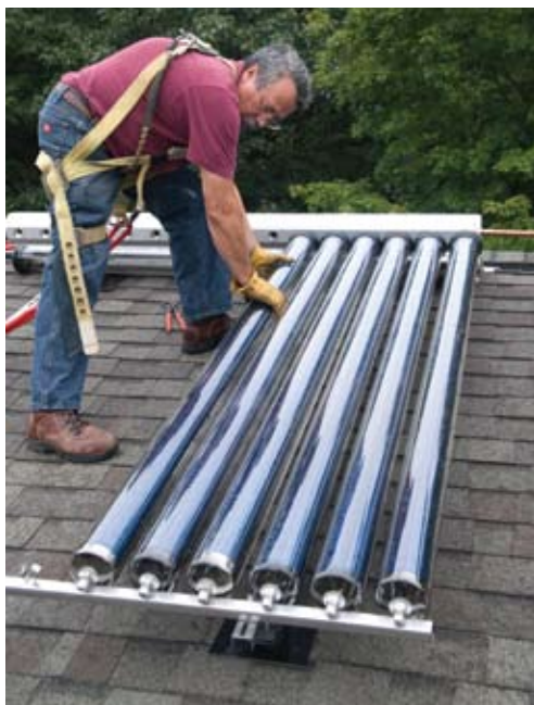
Dave Yates attaches tubes into the Oventrop evacuated tube solar array.
