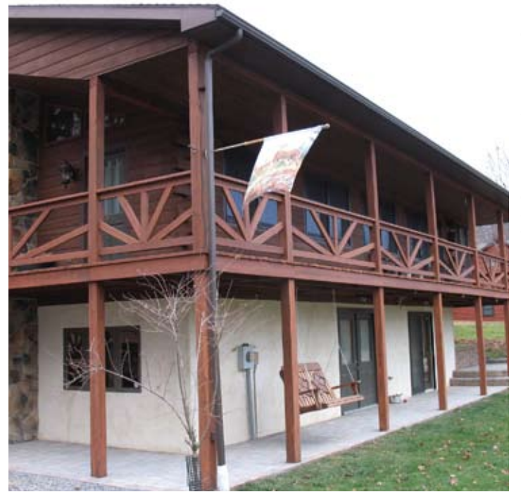
The 2,400-sq.ft., three bedroom log home, located on mountainside property, utilizes an efficient HVAC system with geo-to-radiant heat and a thermal-solar system.
