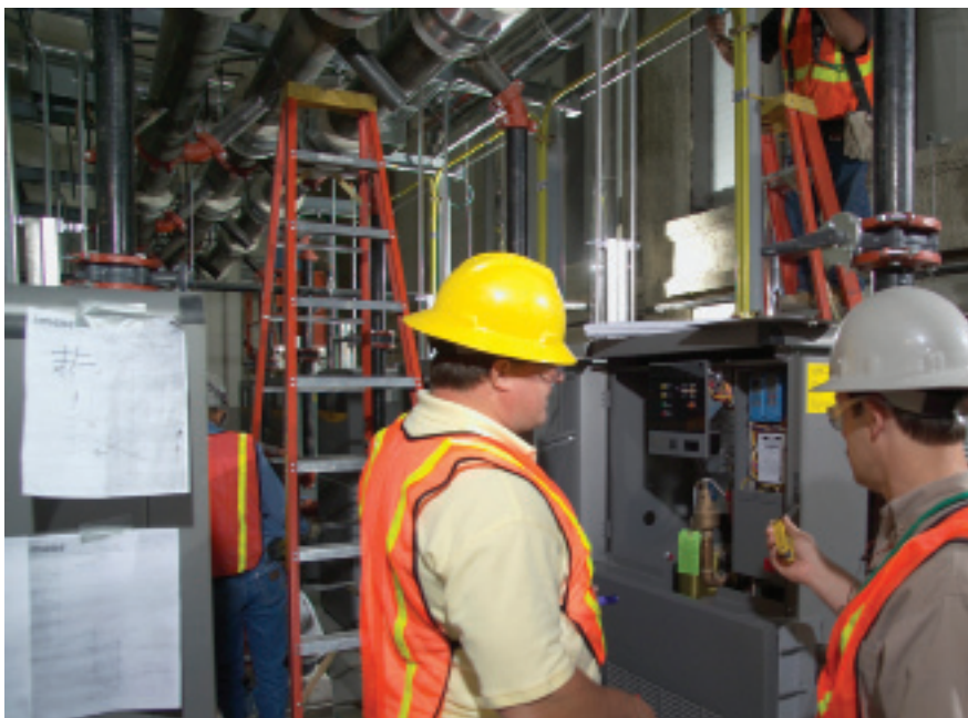
The many Laars Rheos+ boilers are connected in lead-lag fashion to meet all of the facility's space heating needs.
