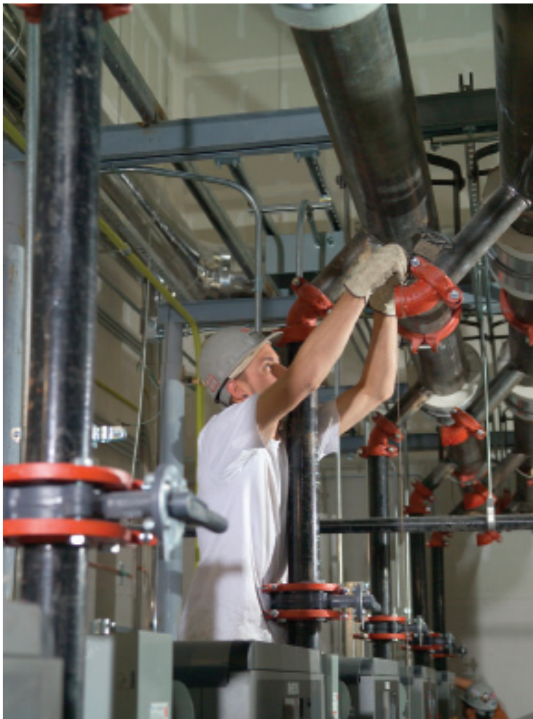
Near-boiler piping is moving quickly towards completion at the Phoenix Convention Center.
