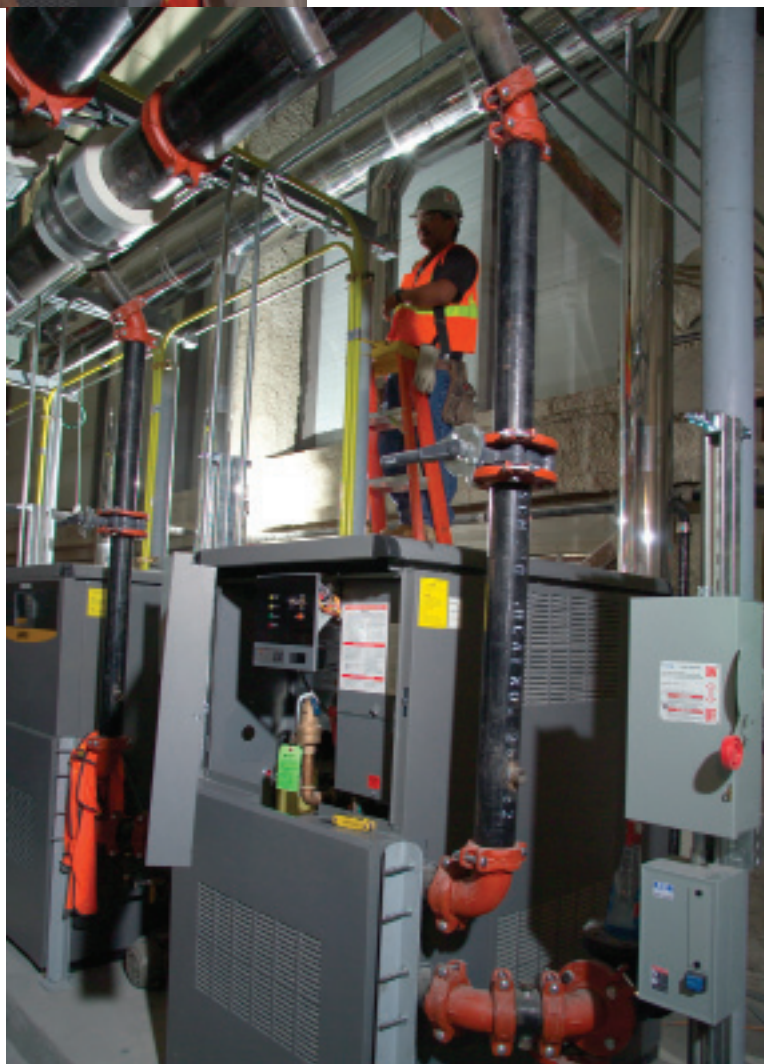
A few of the 10 Laars Rheos+ modulating-condensing boilers.
