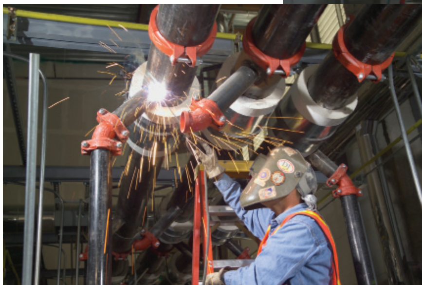
Welders braze joints at one of the boiler headers.
