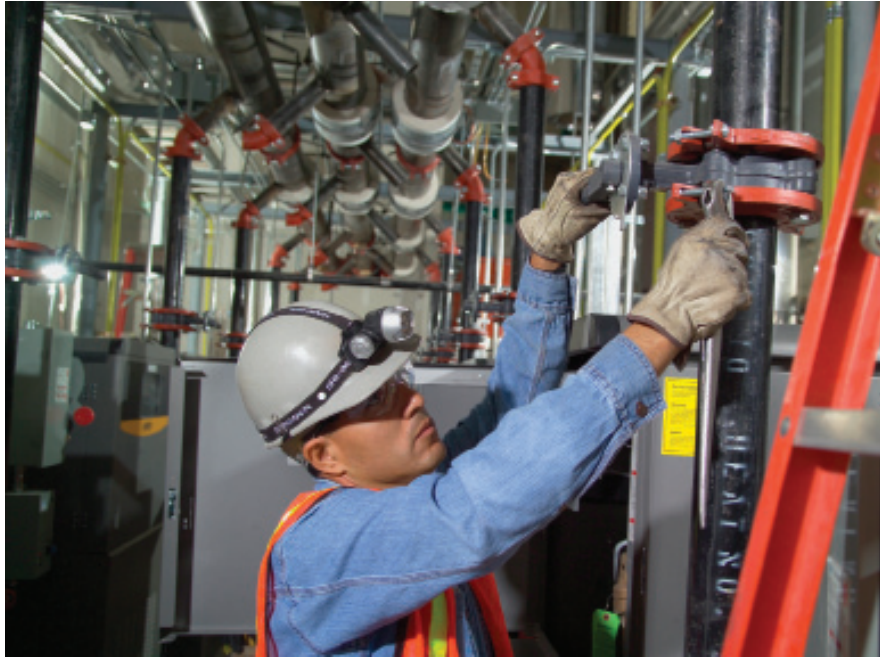
Connections are being finished in preparation for boiler pre-fire.
