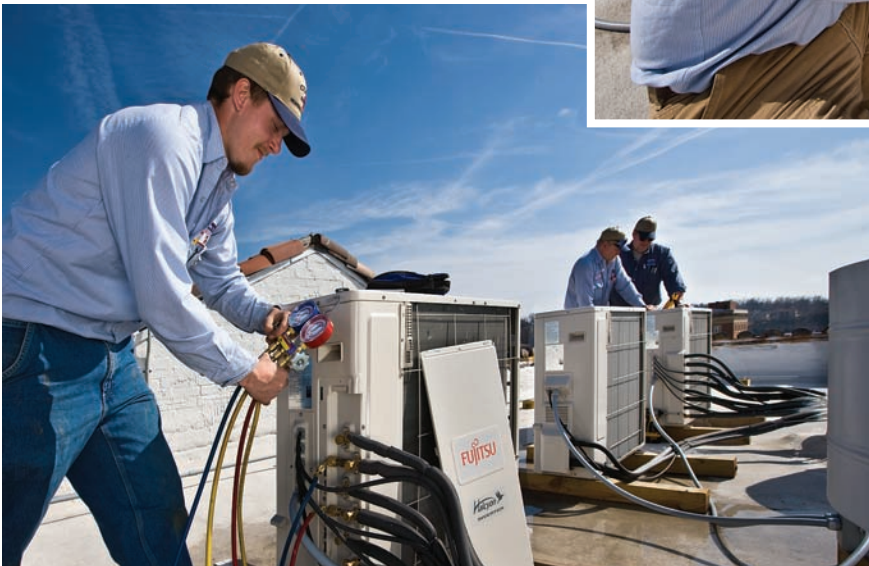
Cash Curtis, service technician, checking R410A refrigerant charge. In the background, David Conner, service manager, and service tech Philip Curtis, owner, checking proper voltage and operation.
