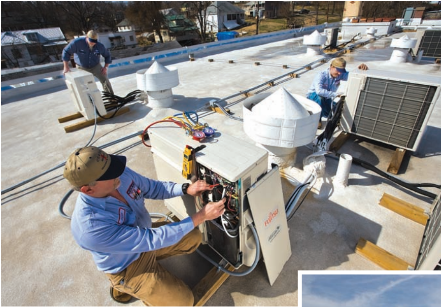
(TOP) David Conner, checking proper voltage as Cash Curtis checks a separate unit while Philip Curtis looks into another unit's refrigeration line set. (RT) David Conner, checking unit out.
