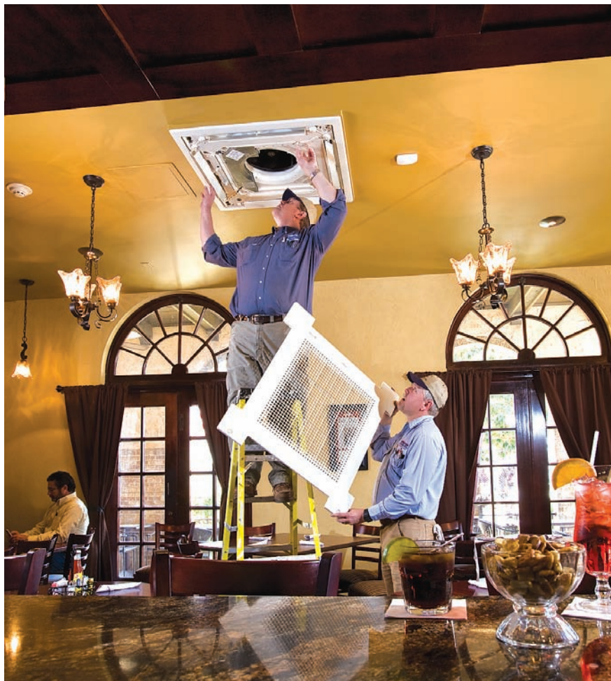
Philip Curtis, owner, on ladder, with David Conner, service manager and tech, in the Hotel's restaurant installing an air intake grill and cover on a ceiling unit.
