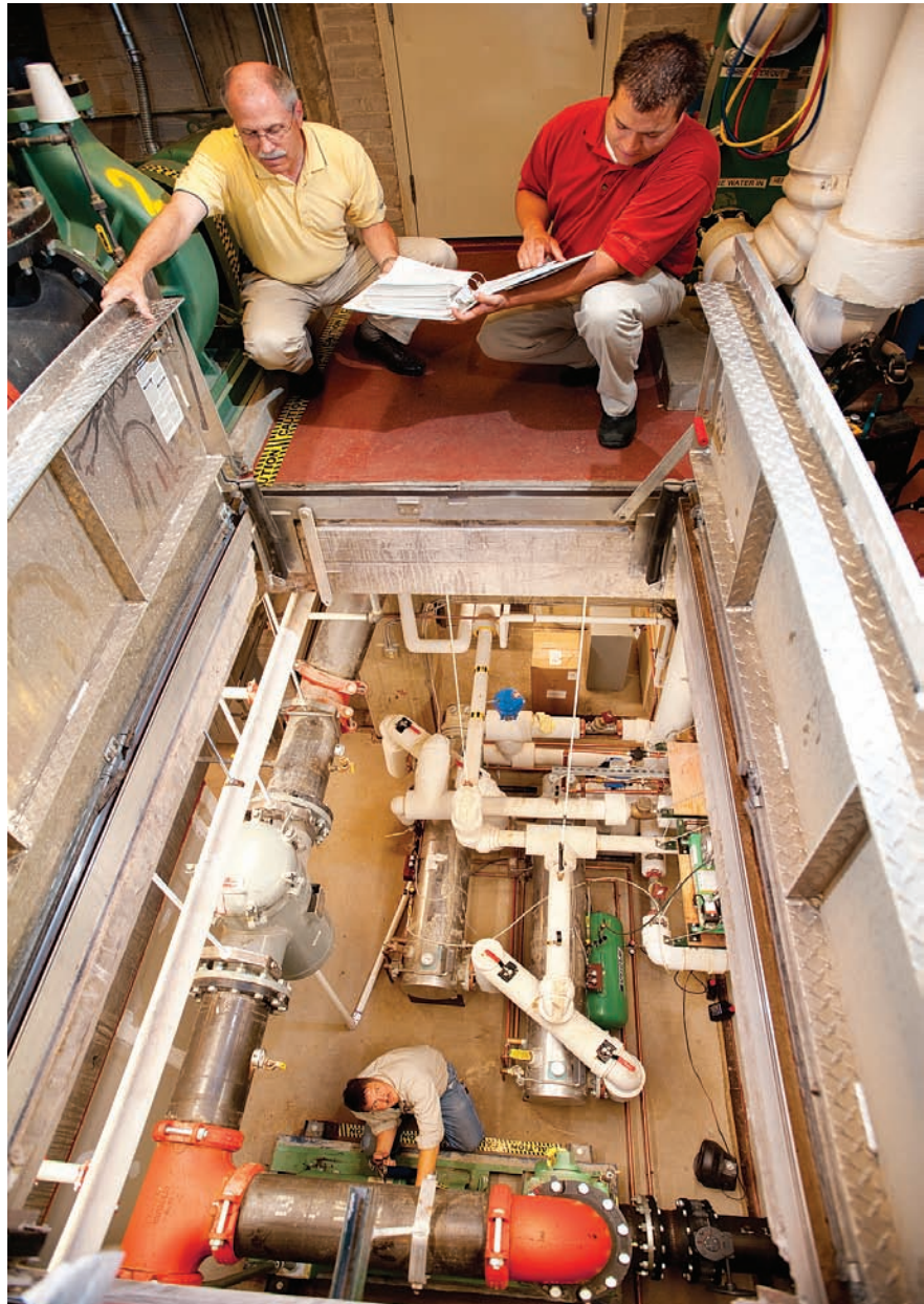
The historic nature of the building left limited options to get all equipment neatly into the main mechanical room, so the creative design/build team used a lower level area to get various needed equipment installed. Access is via the trap doors. The room houses pumps, heat exchangers for domestic hot water, a chemical treatment system, and a lot of piping.
