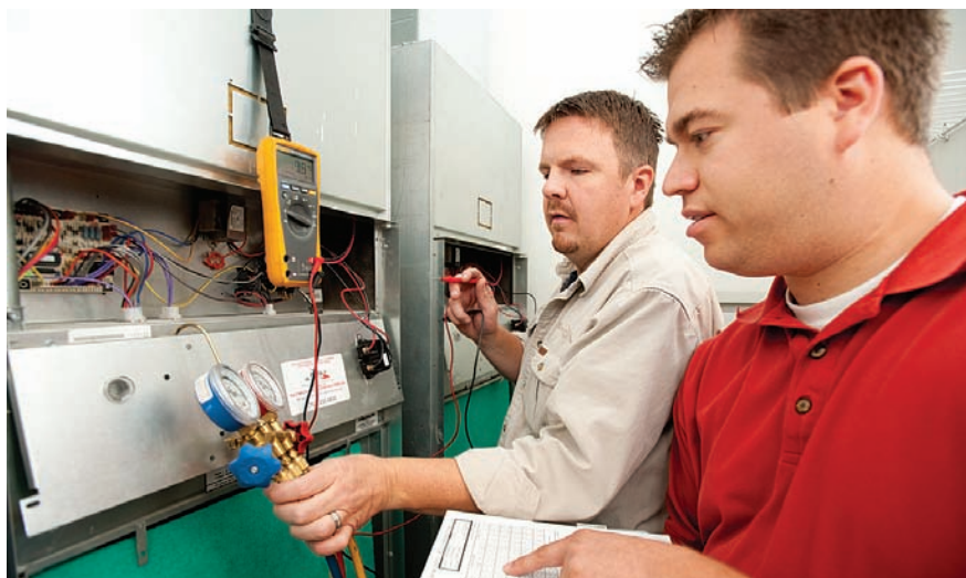
Mechanic Rob Skantz and project engineer Josh Counihan are commissioning the system. Proper commissioning ensures the systems meet the design criteria, and are running properly when the job finishes.
