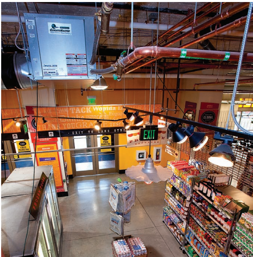
A suspended water-to-air ClimateMaster unit in the retail space was chosen for its super efficiency and the flexibility of being easy to zone. Another factor was the quiet running operation of the equipment.
