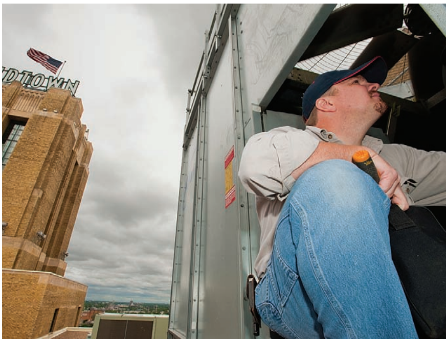
Mechanic Rob Skantz of Horwitz-NSI looks through the service access door of the heat pump system's rather large cooling tower. He could be looking for scale and corrosion or just checking for proper operation.
