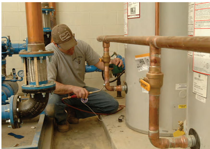
Vrabel plumber Mike Boden sweats a cold water feed line for one of the Bradford White eF water heaters.
