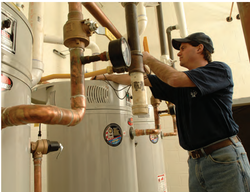
Sean Dewey, jobsite foreman, checks gas pressure feed to the water heaters.
