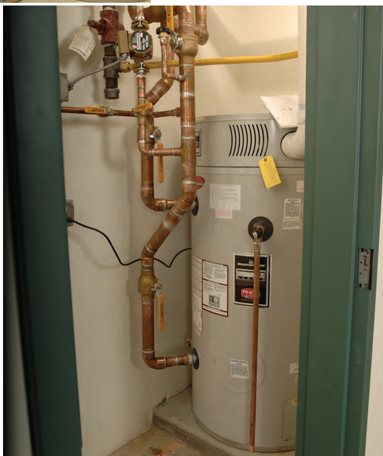
Individual water heaters for each wing reduces the need for water return lines.
