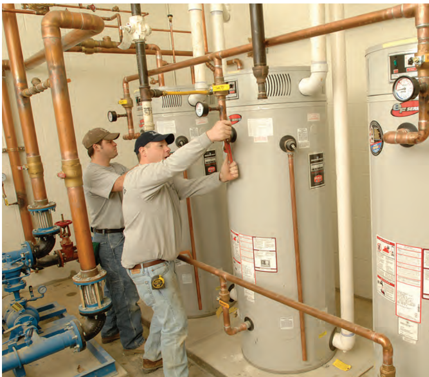
Vrabel plumbers Mike Boden (left) and Mike Gerst tighten nipples for the hot water outlets.
