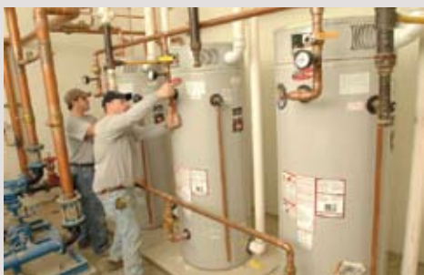
Above, the exterior, showing the four wings of the school. Below, three Bradford White EF water heaters.
