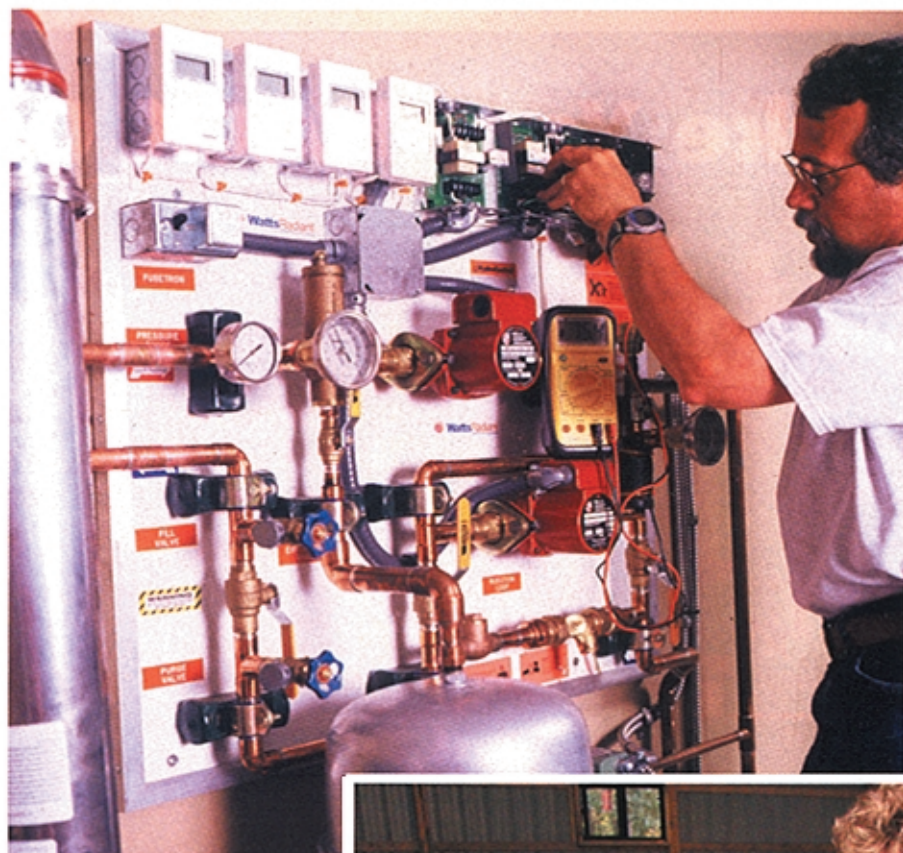
Contractor Dave Yates works at the master board. Injection piping was used to minimize the amount of piping required for the job.
