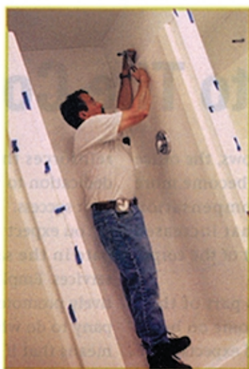
Yates trims out shower faucets as the bath house nears completion.
