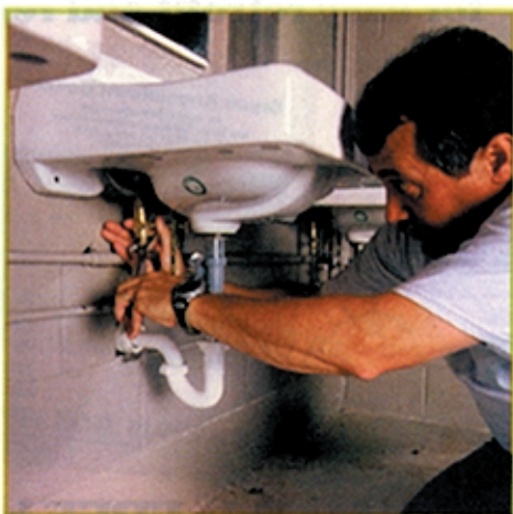
Quick installation of Watts Under-Sink Guardian ASSE 1016 point of use devices will grant scald guard protection for the sink faucets.
