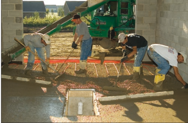
A carwash is a prime candidate for a radiant snowmelting system. Here the concrete is carefully placed over the tubing.
