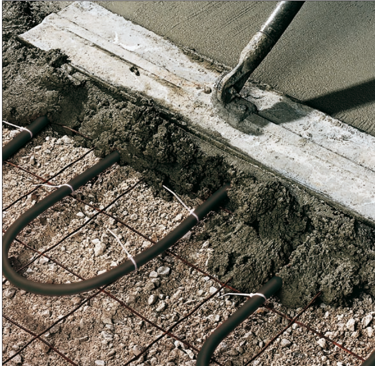
A concrete slab will quickly hide the network of radiant heat tubing below.
