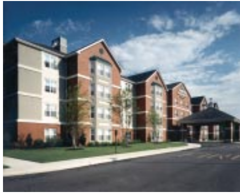
The long-term ownership objectives for the Elizabethtown (PA) public library (far left) and the Homewood Suites in Wilmington, DE, drove the selection of the buildings' materials.
