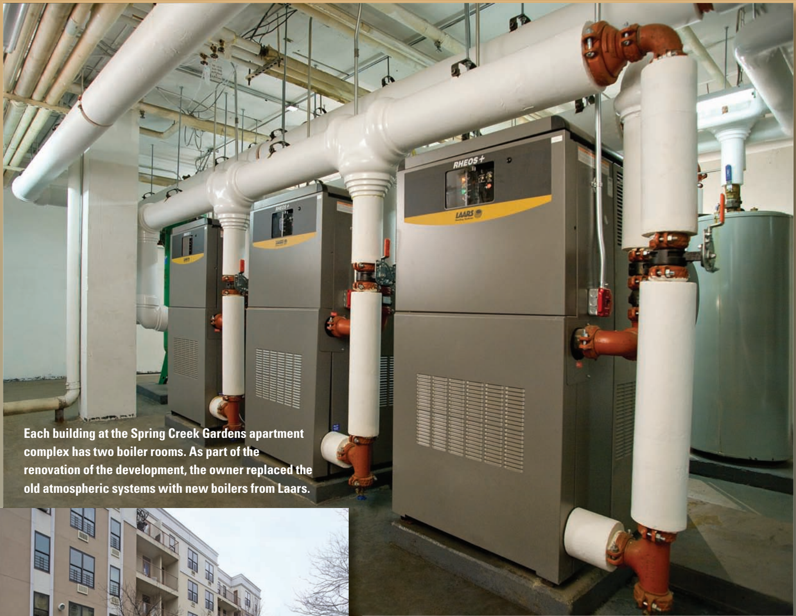
◀ Spring Creek Gardens, Brooklyn, NY, was built in 1986. The low-rise apartment complex of affordable rental units was renovated top-to-bottom. The original heating equipment was replaced with high-efficiency boilers for heating and domestic hot water.
