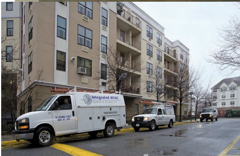
Each building at the Spring Creek Gardens apartment complex has two boiler rooms. As part of the renovation of the development, the owner replaced the old atmospheric systems with new boilers from Laars.
