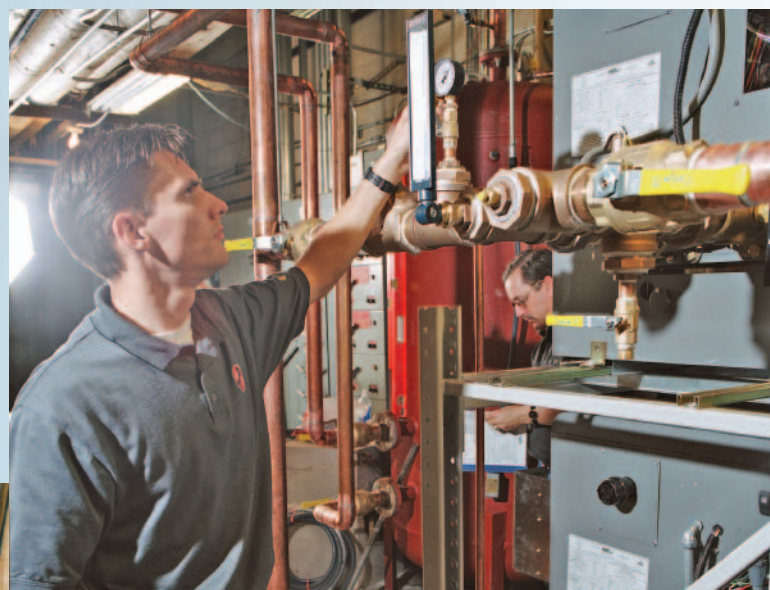
Jim Beatty, service technician, inspects the Laars equipment during installation.
