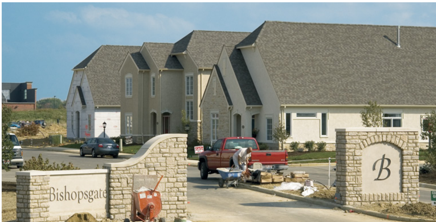
The Bishopsgate condominium development in Ohio is relying on radiant heating throughout
