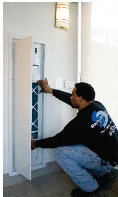
A ClimateMaster technician checks the filter of a vertical stack unit.
