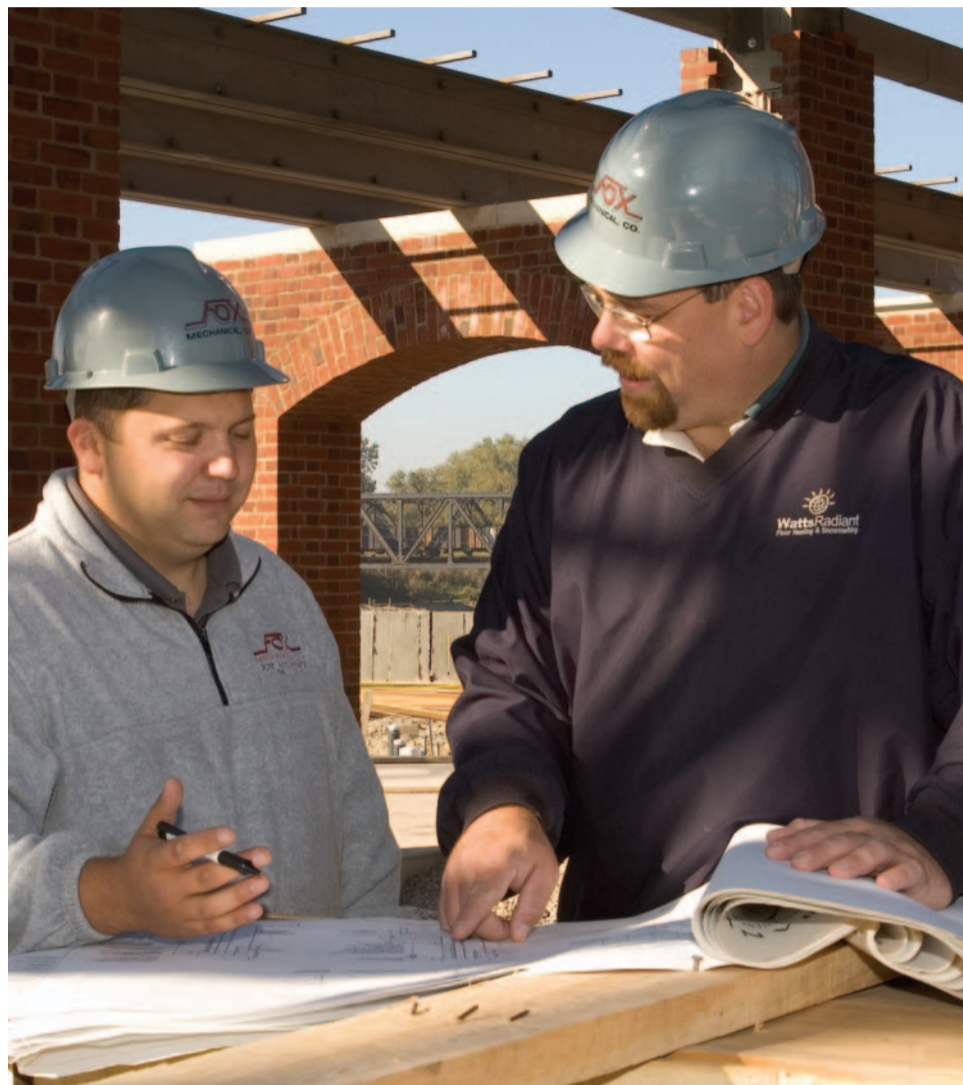
Planning Ahead For Year-Round Comfort: Andy Fox, vice president, Fox Mechanical (left), and Hanse Cromer, manufacturer's rep with Steffens-Shultz, discuss the layout of the radiant heat grid for the riverside pavilion at Northbank Park in Columbus, Ohio. For the full story, see page 20.
