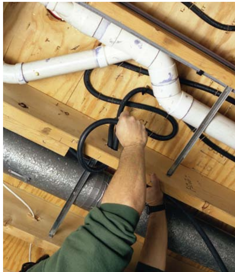
Yates prefers Onix tubing for any radiant retrofit work, especially for staple-up applications. The tubing is swerved and connected to miss protruding nails.
