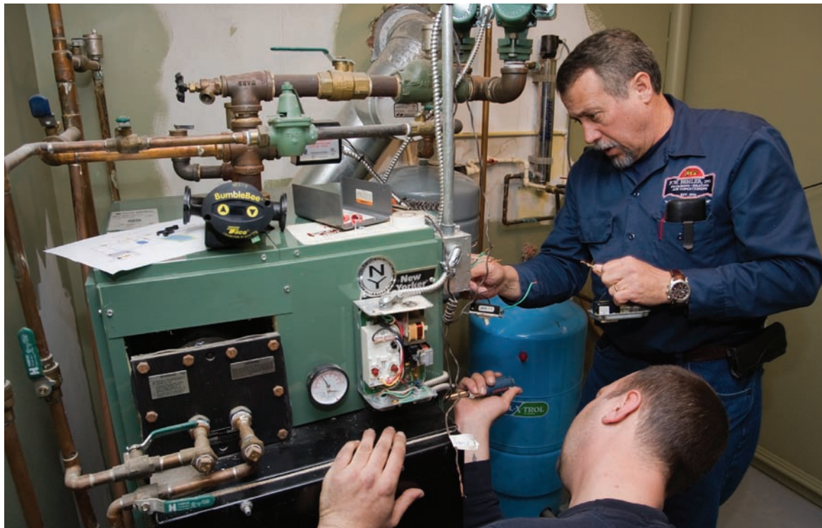
Top: Dave Yates, owner of York, PA-based F.W. Behler, Inc. and technician Larry Lawrence, begin disassembly of the original oil-fired New Yorker boiler at the beginning of the hydronic system retrofit. Above: Disassembly of the oversized but functional boiler was completed with care. The homeowner sold the boiler to a neighbor whose old farmhouse is much larger and with a boiler badly in need of replacement.
