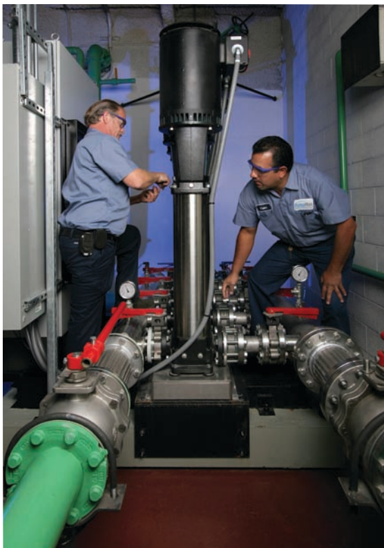
The new four-pump pressure-boosting system.
