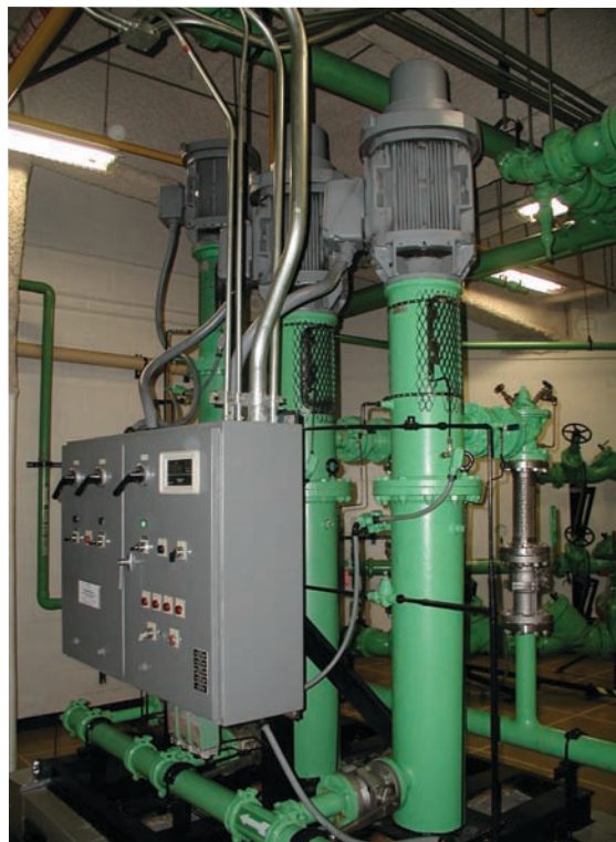
The high zone's original three-pump pressure-boosting system.
