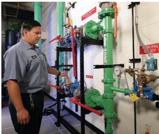
The low zone's new pressure-regulation station.
