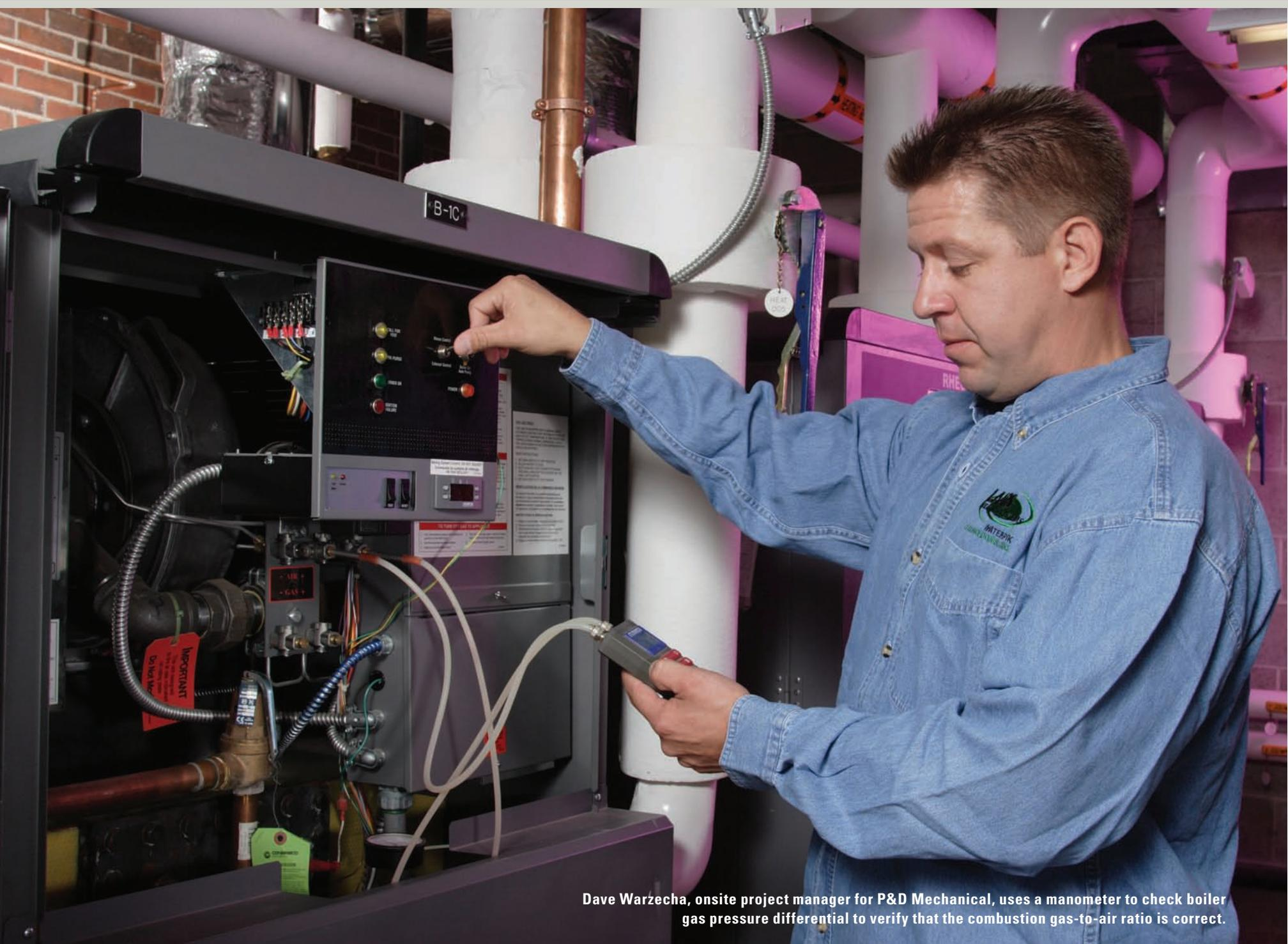
Dave Warzecha, onsite project manager for P&D Mechanical, uses a manometer to check boiler gas pressure differential to verify that the combustion gas-to-air ratio is correct.
