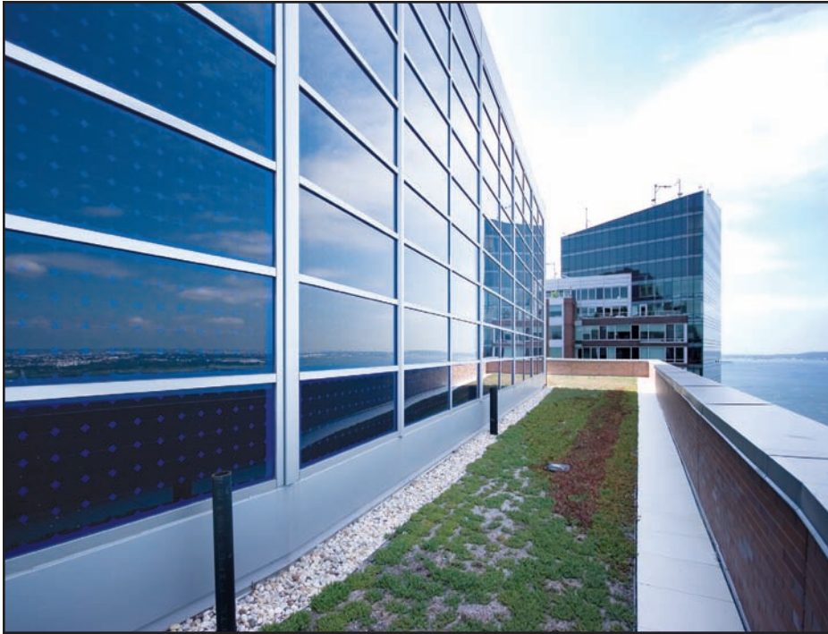
The green spaces on the roof of Millennium Tower contribute to the building's LEED® pursuit.
