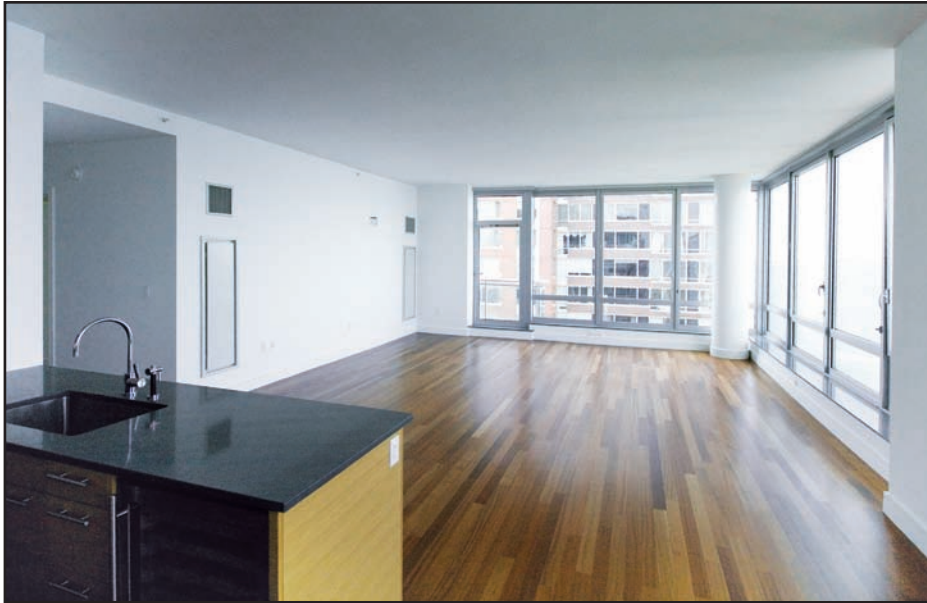
View of a condominium living room shows how neatly the central system's water-to-air vertical units are integrated discreetly.
