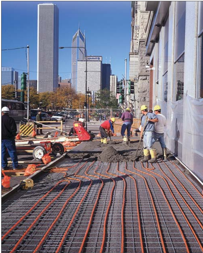
Snowmelting can be accomplished with the efficient circulation of a low temperature glycol/water solution.
