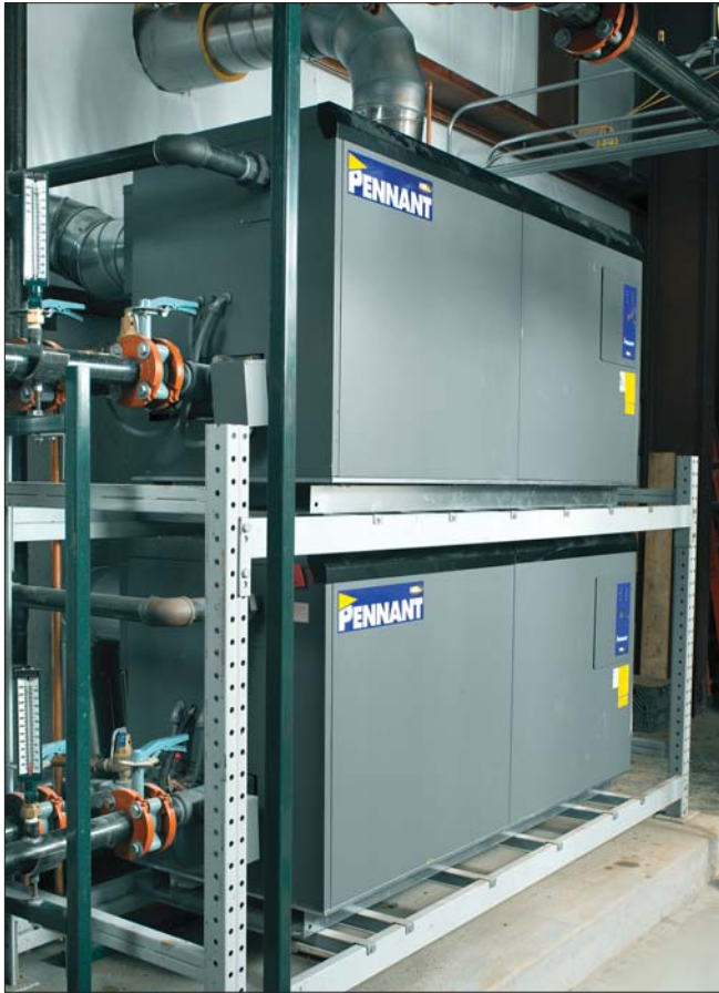
Low NOx, high-efficiency boilers can be stacked to economize on mechanical room floor space and for ease of service. (Photo courtesy of Laars.)
