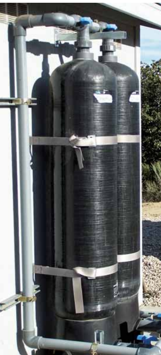
Watts OneFlow system prevents scale problems throughout the winery's distribution system.
